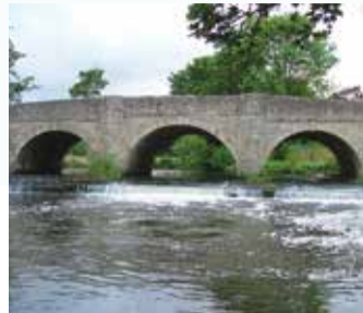
Old stone arched bridge crossing the River Teme at Leintwardine
